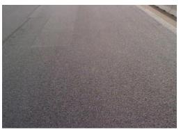
that water and salt during the time in which it freezes and thaws, remains in the asphalt cavities and slowly begins to destroy the asphalt. The vehicles that then roll over these areas tear up bit by bit the loose asphalt and accelerate the deterioration process (Gunter, 2012; Willoughby, 2003).
