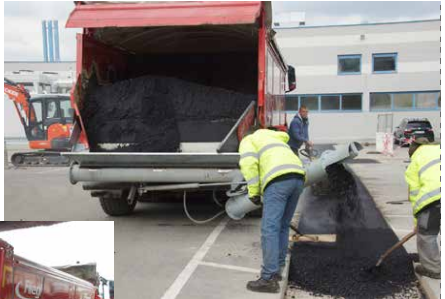
← "Wiesel" distribution screw can be simply attached / retrofitted
